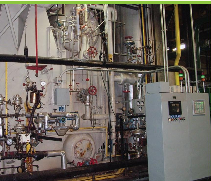
The steam system at Goodyear's Union City plant is served by four dual fueled (natural gas and No. 6 fuel oil) boilers, such as the 60,000 lbs/hr boiler pictured above.
