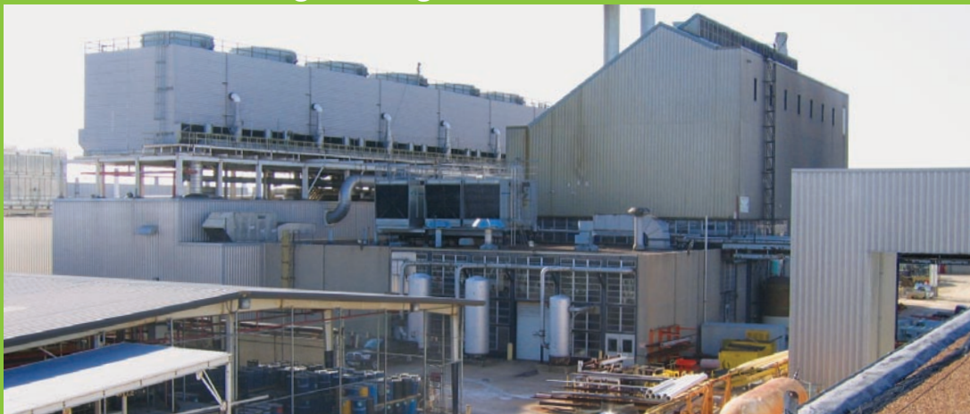
The powerhouse at Chrysler's St. Louis Assembly Complex provides steam, chilled water, and compressed air to both the north and south plants.
